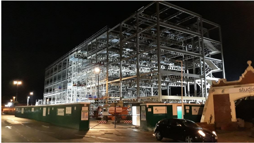
Teville Gate House Construction 12/12/2019
